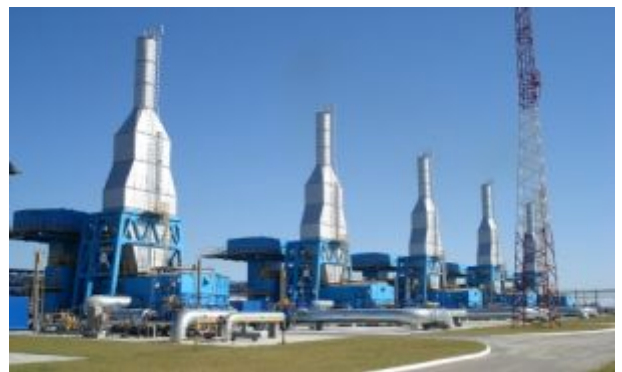
GPA-C-16S with UGT 15000 gas turbine at Novopetrovskaya compressor station, Yamburg, Russia
