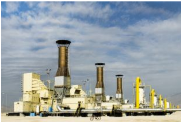
GPA-C-25S with UGT 25000 gas turbine at Potaveh compressor station, Iran
