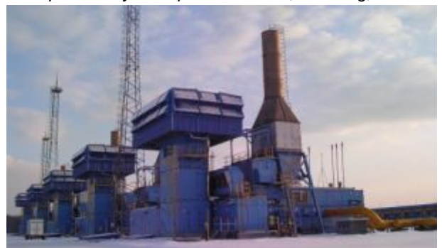
GPA-C-16S with UGT 15000 gas turbine at Slonim compressor station, Belarus
