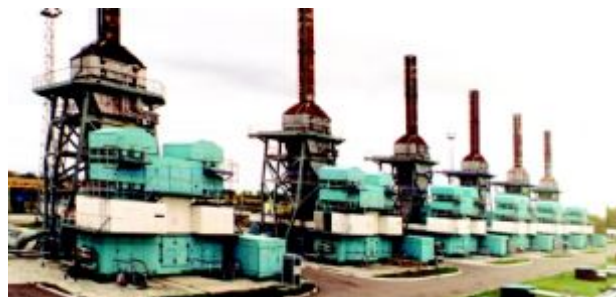
GPA-C-6,3 with DT71 gas turbine at Dikanka compressor station, Ukraine.
