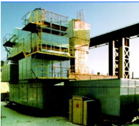
Gas pumping unit GPA-C-6,3S with DT71 gas turbine
