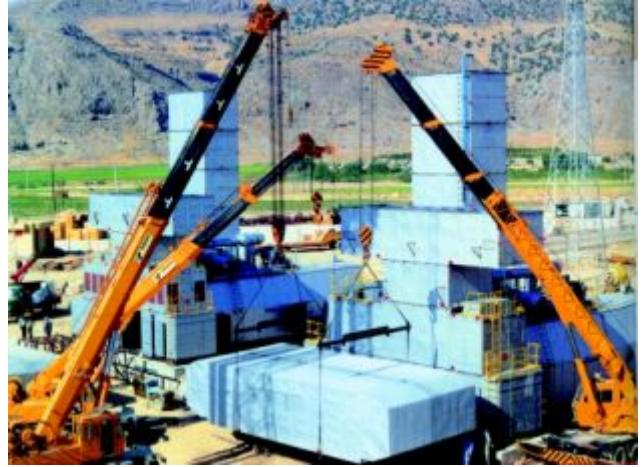
Compressor station with UGT 16000 gas turbines construction in Iran
