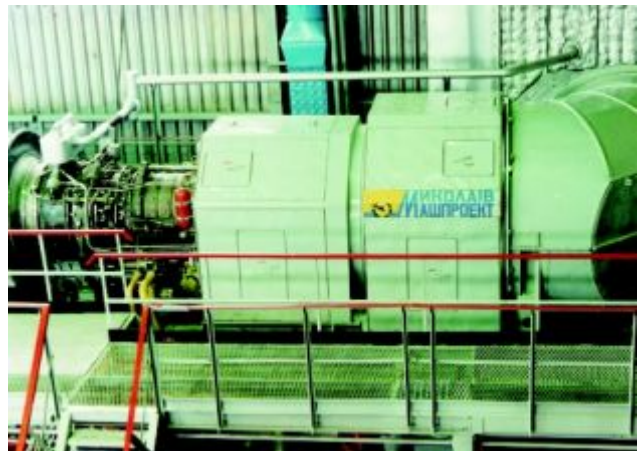
Modernized gas pumping unit GPA-25/76 in the engine room of Sofievskya compressor station, Ukraine
