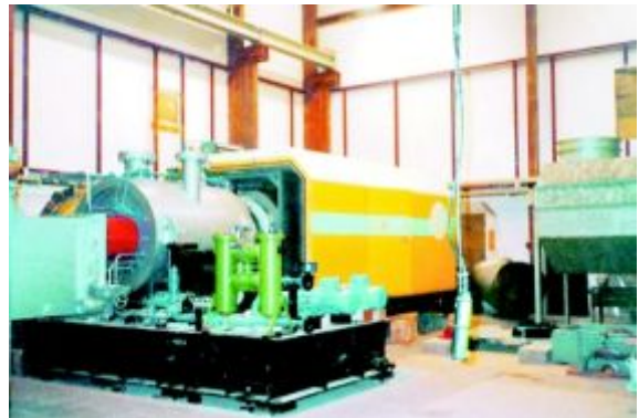
Gas pumping unit driven by DE76E at Stramberk underground gas storage engine room
