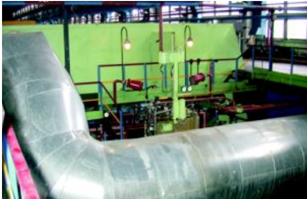
DN70L gas turbine in the modernized GTK-10-4 gas pumping unit at compressor station Kirovogradskaya, Ukraine
