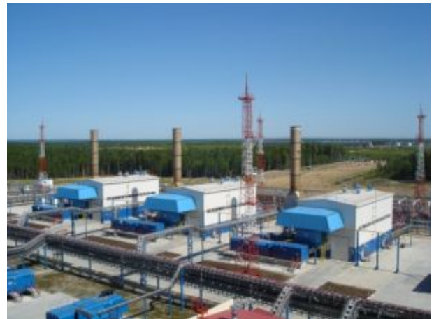
URAL GPA-25S with UGT 25000 gas turbine at Tayozhnaya compressor station, Yamburg, Russia
