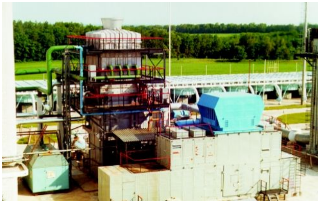
Gas pumping unit GPU-16K at Stavishchenskaya compressor station, Ukraine
